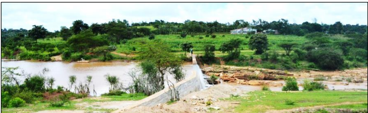
Figure 1: Photo of sand dam in Kithyululu, Kenya
